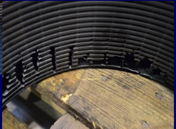
Wrong Material selection
